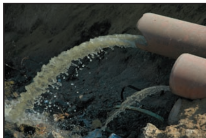
Raw sewage, Gaza Strip
